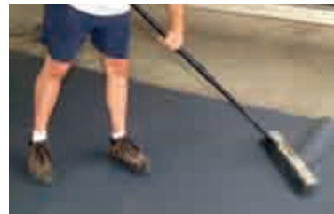
Push out any air with a broom
