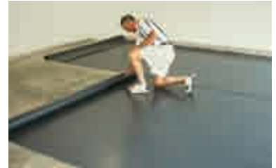
Roll out flooring front-to-back
