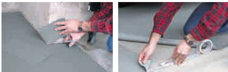
For optional taping of front edge use 2-sided tape or 3M® brand 80 Rubber & Vinyl Spray Adhesive
