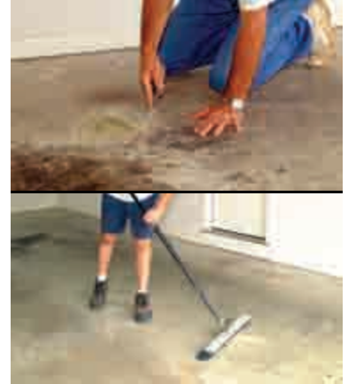
Clean floor before applying flooring
