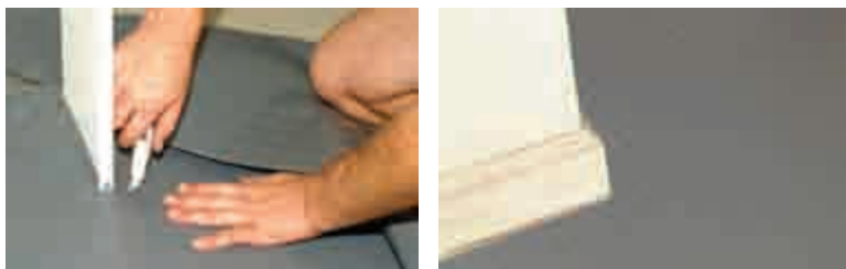
Trim carefully around edges leaving 1/4" gap
